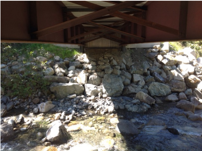
Left Bank Abutment when facing downstream
