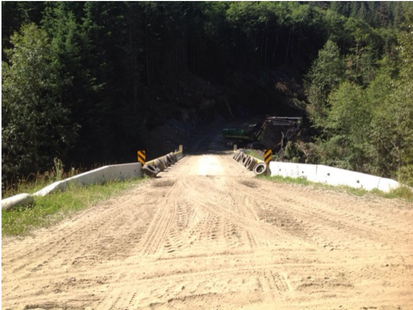
Approach from Right Bank when facing downstream
