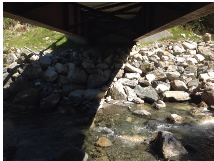
Right Bank Abutment when facing downstream
